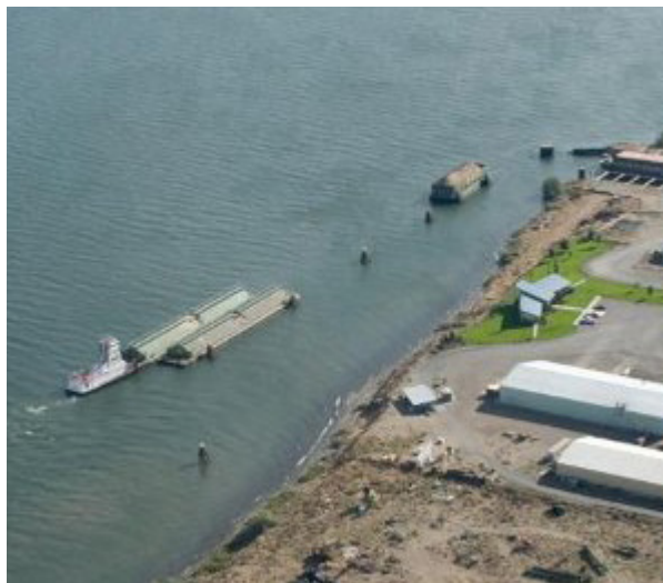
Boardman Port (Tidewater Barge)
