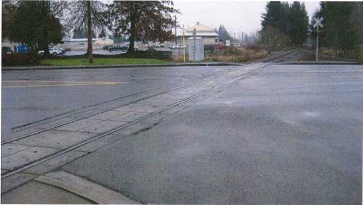
Pre-construction conditions at grade crossing: main line
