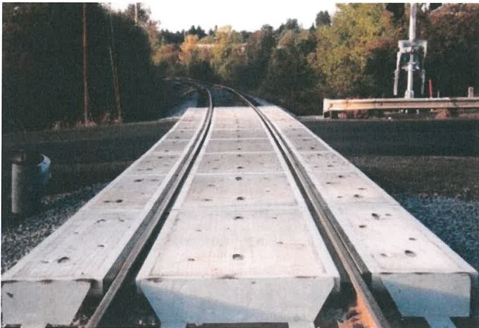
Example of expected crossing conditions post-construction with concrete panel crossing surface
