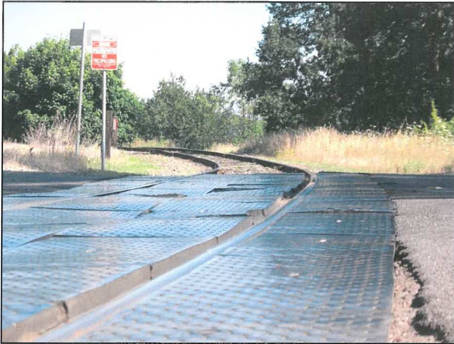
Example of expected crossing conditions post-construction with concrete panel crossing surface
