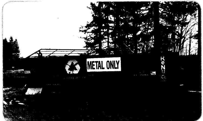
Separation of materials with economic value, such as metals, at a construction site can help reduce project costs.
