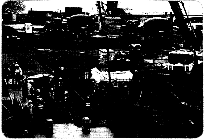
Construction of new transfer stations, such as the Bow Lake station, is financed using general obligation bonds.
