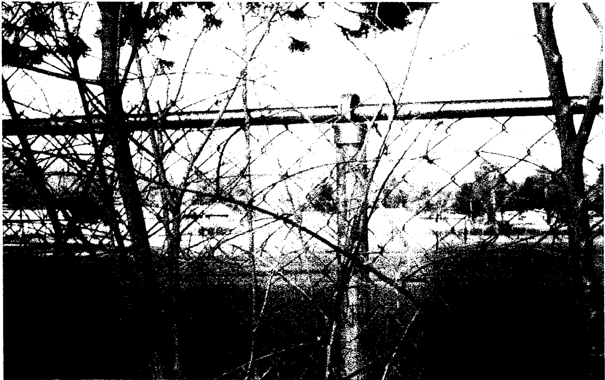
The school district maintenance department is constantly repairing damage to the fence, which has been cut to gain access to the playground from the railroad right-of-way.
