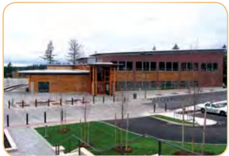
With technical and financial assistance from the division's green building program, the City of Sammamish built a new city hall that showcases environmentally sustainable building and construction.
