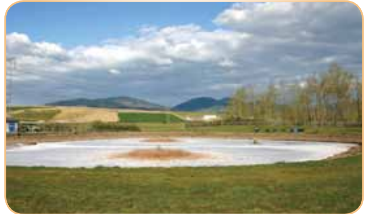
Leachate from the landfill is pretreated in an aeration pond before being sent to a wastewater treatment plant.
