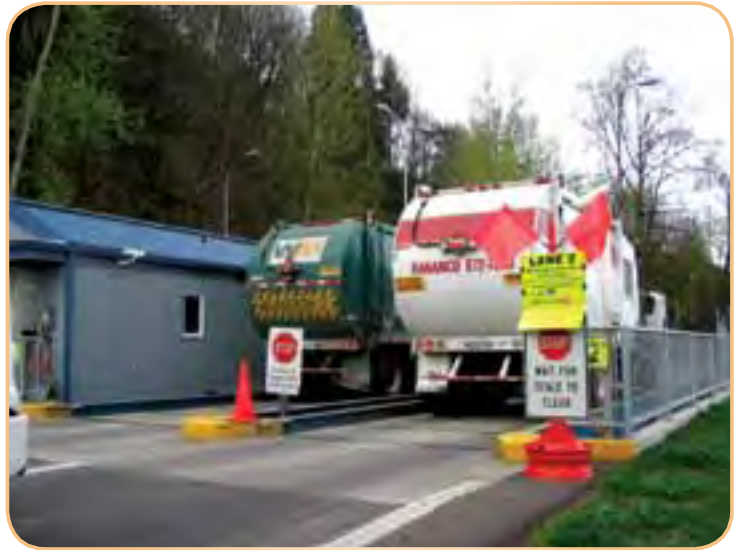
Two outbound scales at the Algona Transfer Station help keep traffic moving through the station.
