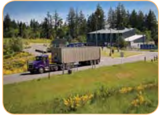
The Vashon Transfer/Recycling Station replaced the Vashon landfill in 1999.
