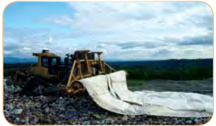
The Tarp-O-Matic covers the working face of the landfill at the end of each day.
