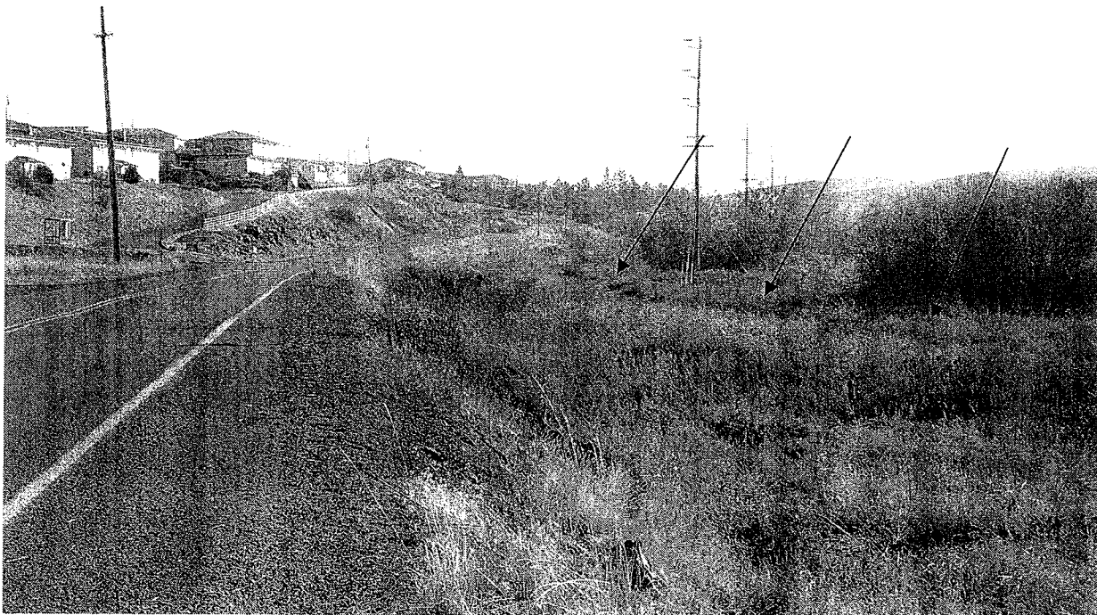
Narrow shoulders would require extensive fill in wetlands adjacent to roadway. Arrows indicate proposed path location on abandoned rail bed. Buildings at upper left are low cost housing units served by the project.
