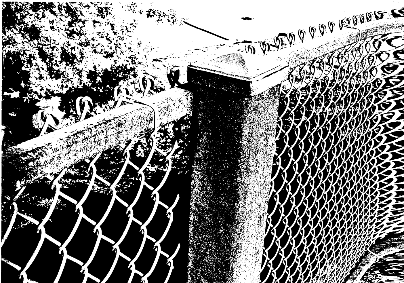
This is a fence located in Wenatchee Wash., that the Proposed fence in Skykomish is designed from
