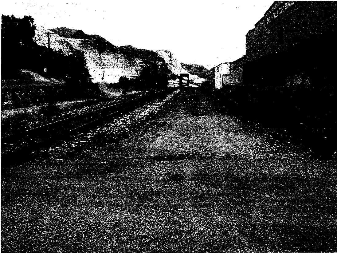
CHESTNUT STREET RAILROAD CROSSING Looking Northerly
