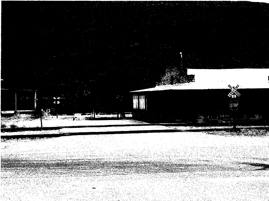
CHESTNUT STREET RAILROAD CROSSING Looking Easterly
