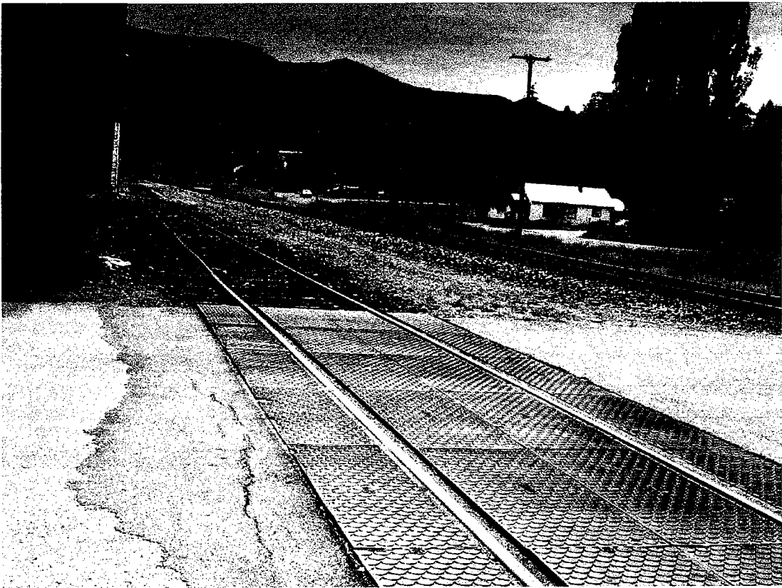
CHESTNUT STREET RAILROAD CROSSING Looking Southerly
