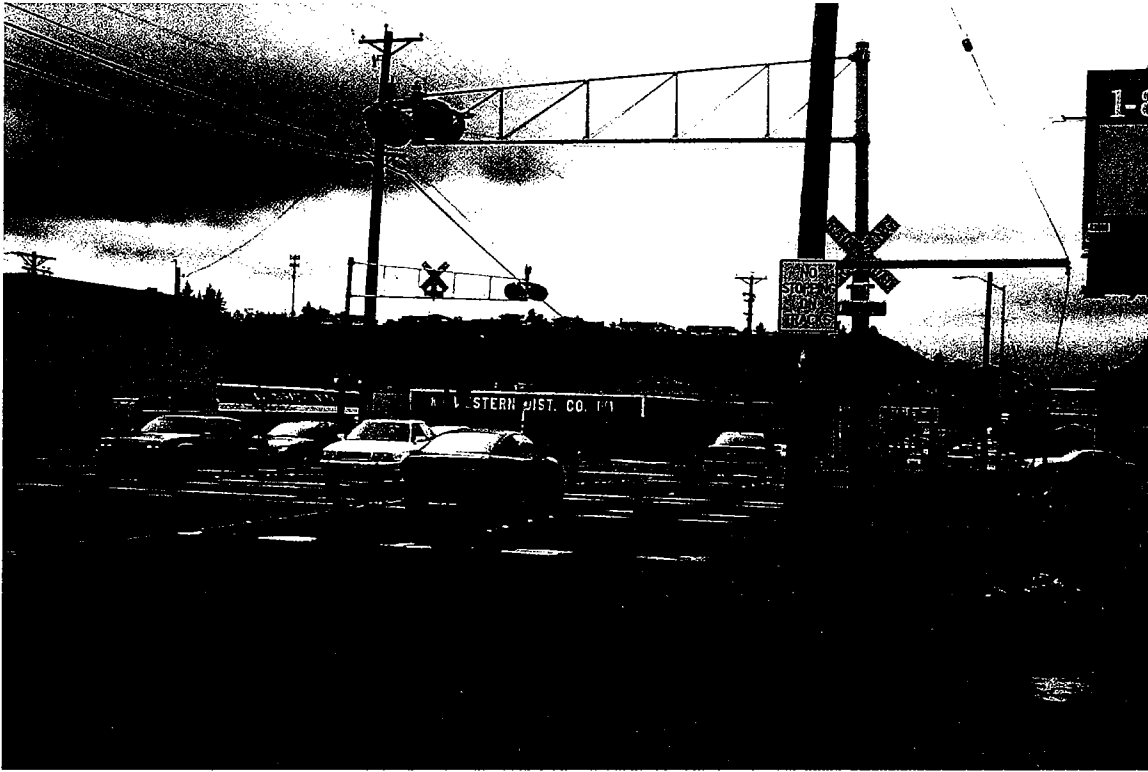
South 56 th Street – 085393V Sound Transit Commuter Rail (former BNSF mainline track)
