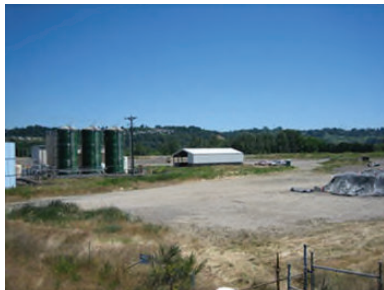
View East of the Tideflats Station
