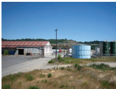
View Northeast of the Tideflats Station
