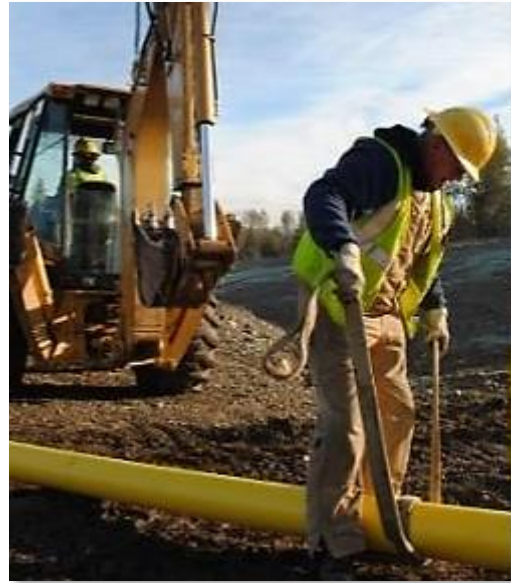
Figure 8. Natural Gas Pipe Installation
