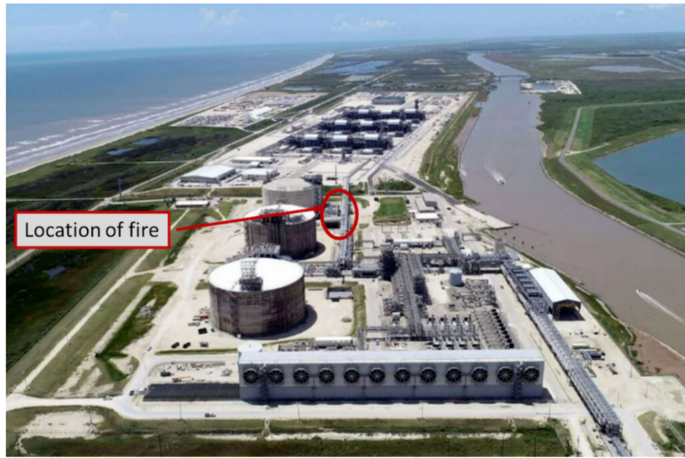
Freeport LNG complex, now a leading shipper of gas to Europe, is set to open partially in September after a June 8 pipeline fire, but full operation may not occur until late 2022. Image: RBN Energy
