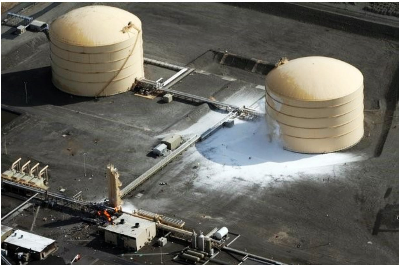
Aerial view taken shortly after the failure. Fires still burning. Perlite insulation leakage from the penetrated outer LNG-1 storage tank. Control room lower left.
