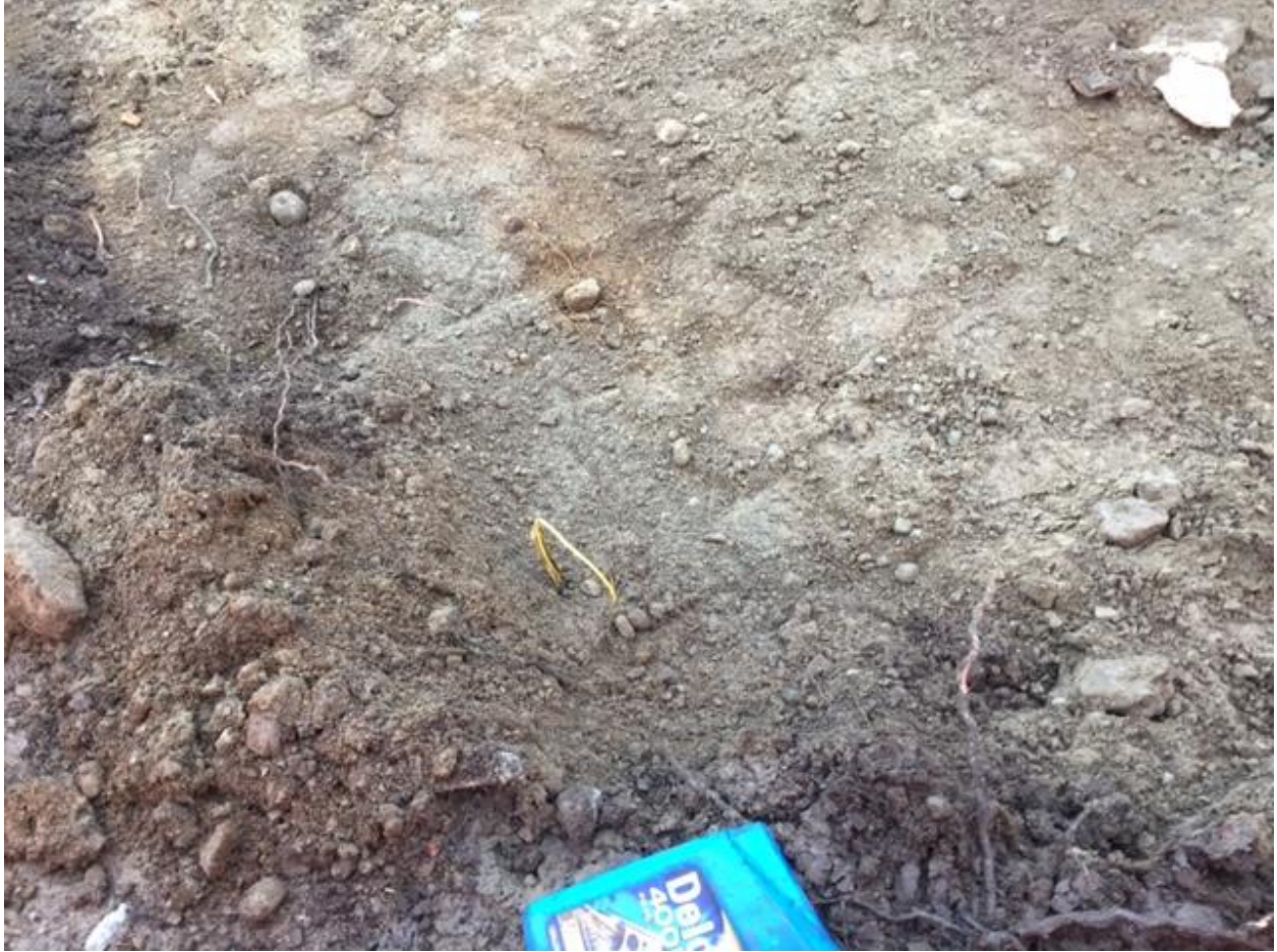
Gas Stub Marker that had been damaged and covered
