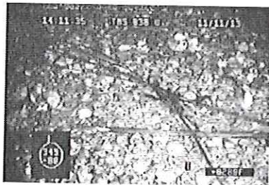
Figure 5 - Parted Cable End Eastern Side
