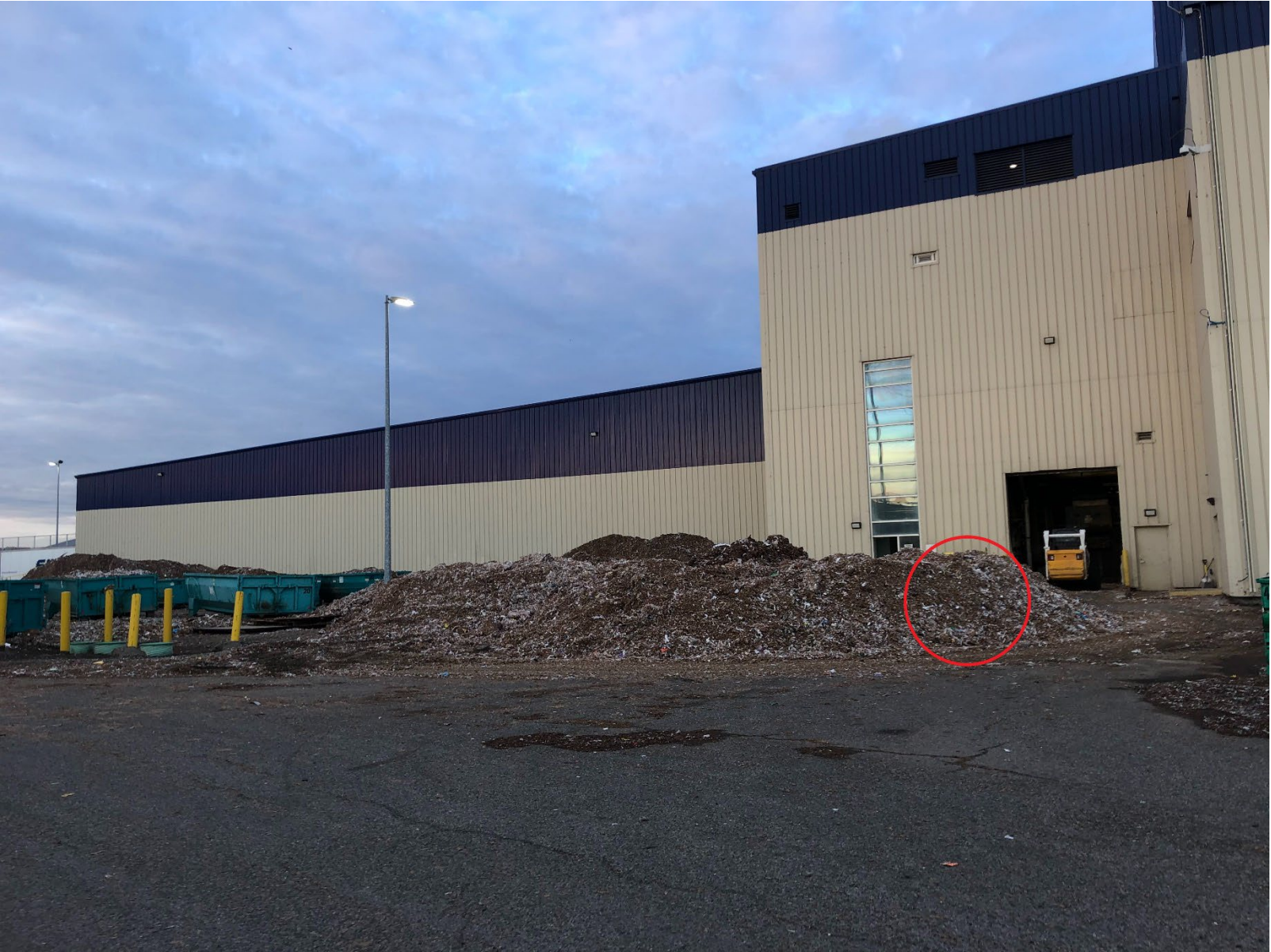
May 21, 2021- Red circle indicates where the fire hydrant usually is before it was covered with OCC Rejects.
