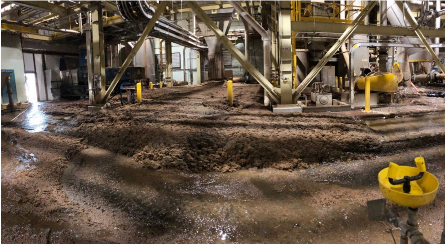
Effluent rejects consisting of stock and water. This is a typical scenario during an annual shut down.
