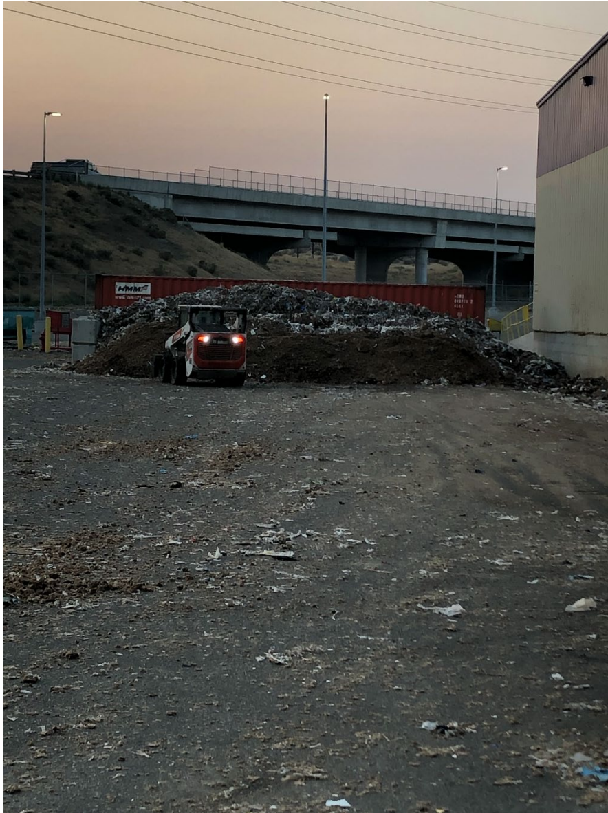
September 19, 2021- Jammies has added their Conex and eliminated the piles and dumpsters in front of the facility.
