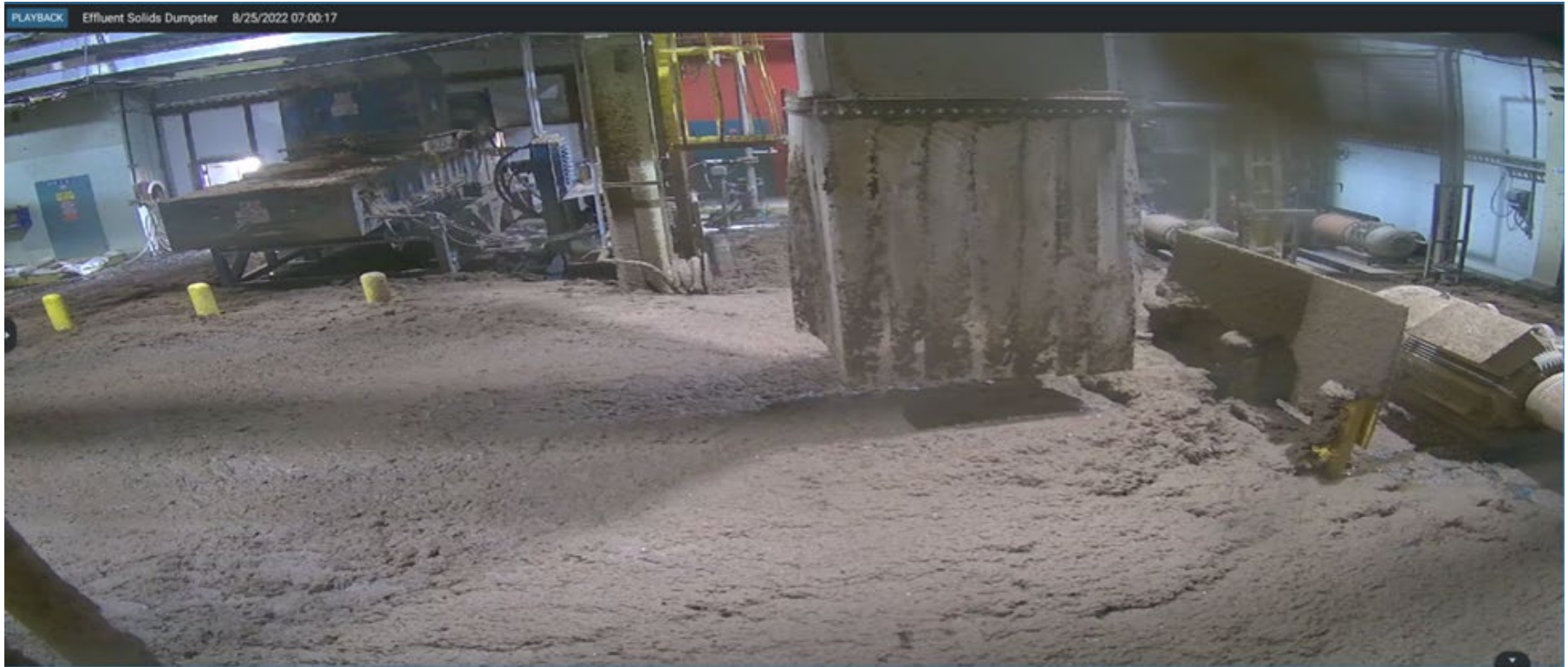
Effluent rejects consisting of stock and water. This is what we expect during an annual shut down.
