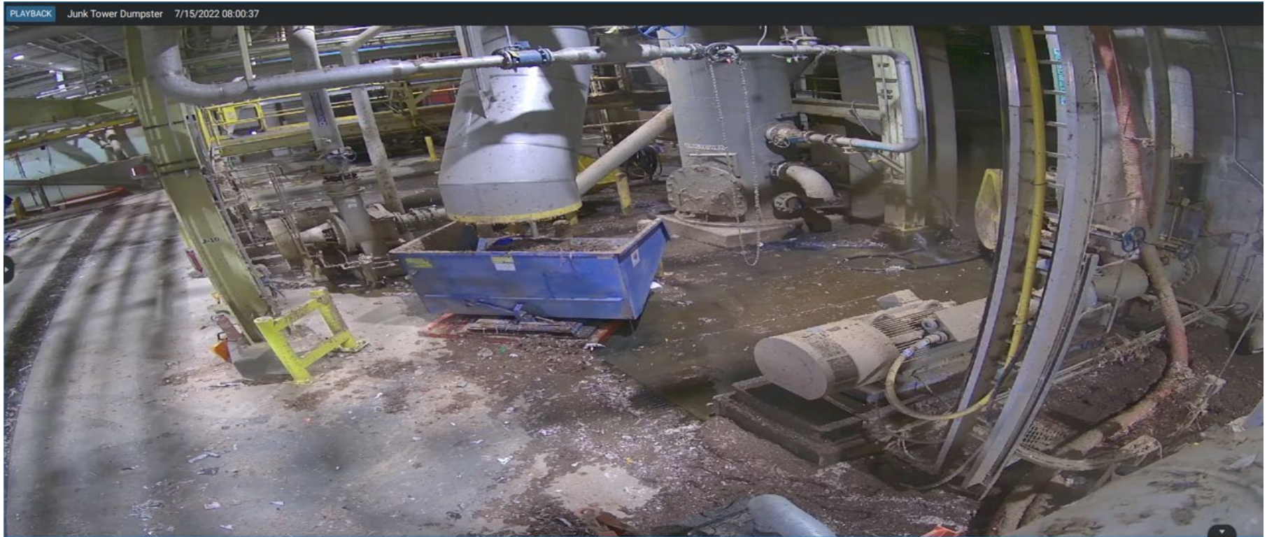
OCC Rejects from the Junk Tower Dumpster. These rejects are made up of heavy metals and wet strength cardboard. They contain between 40-50% water.
