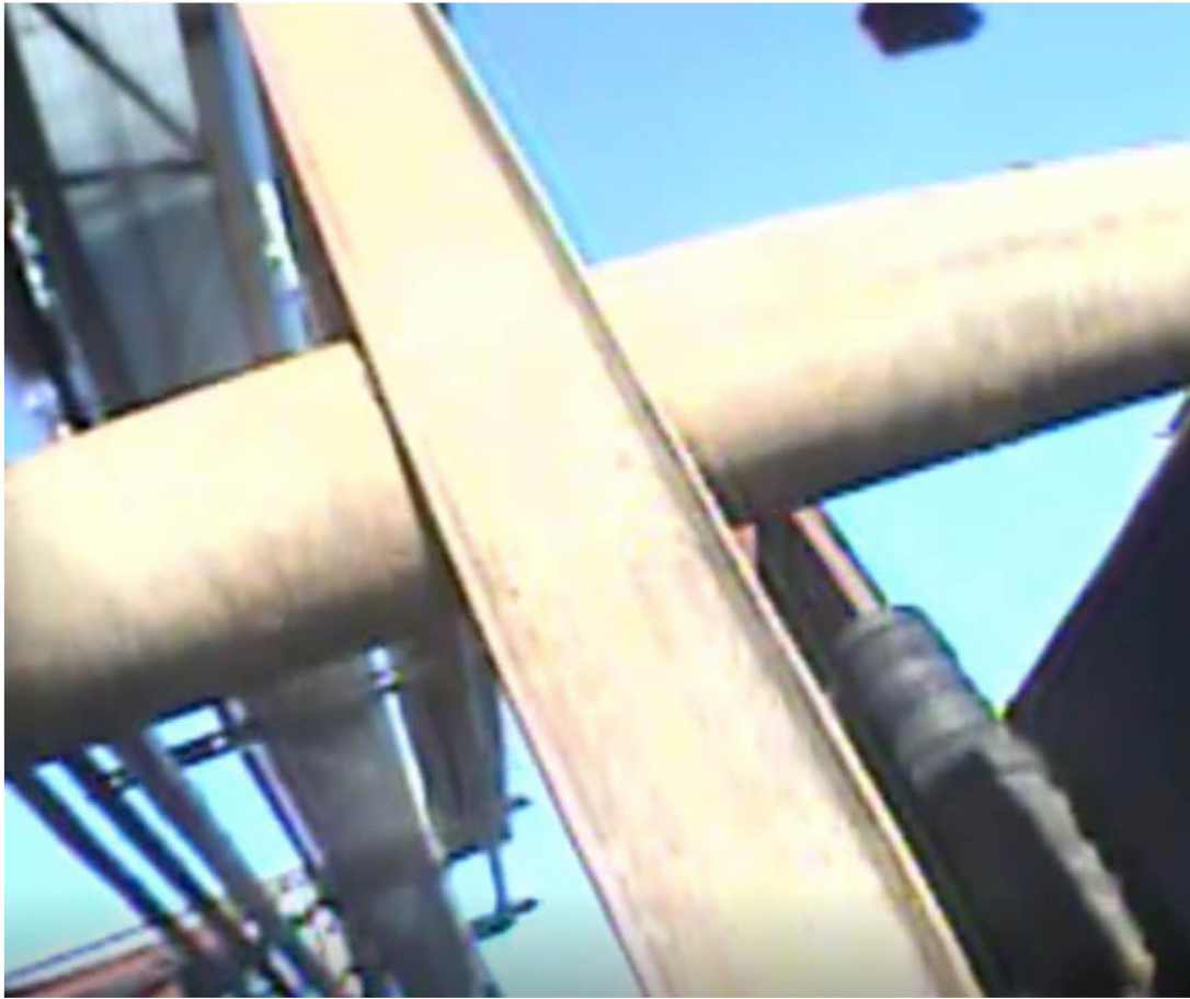
Figure 12- Above water view of vertical channel support welded into horizontal support
