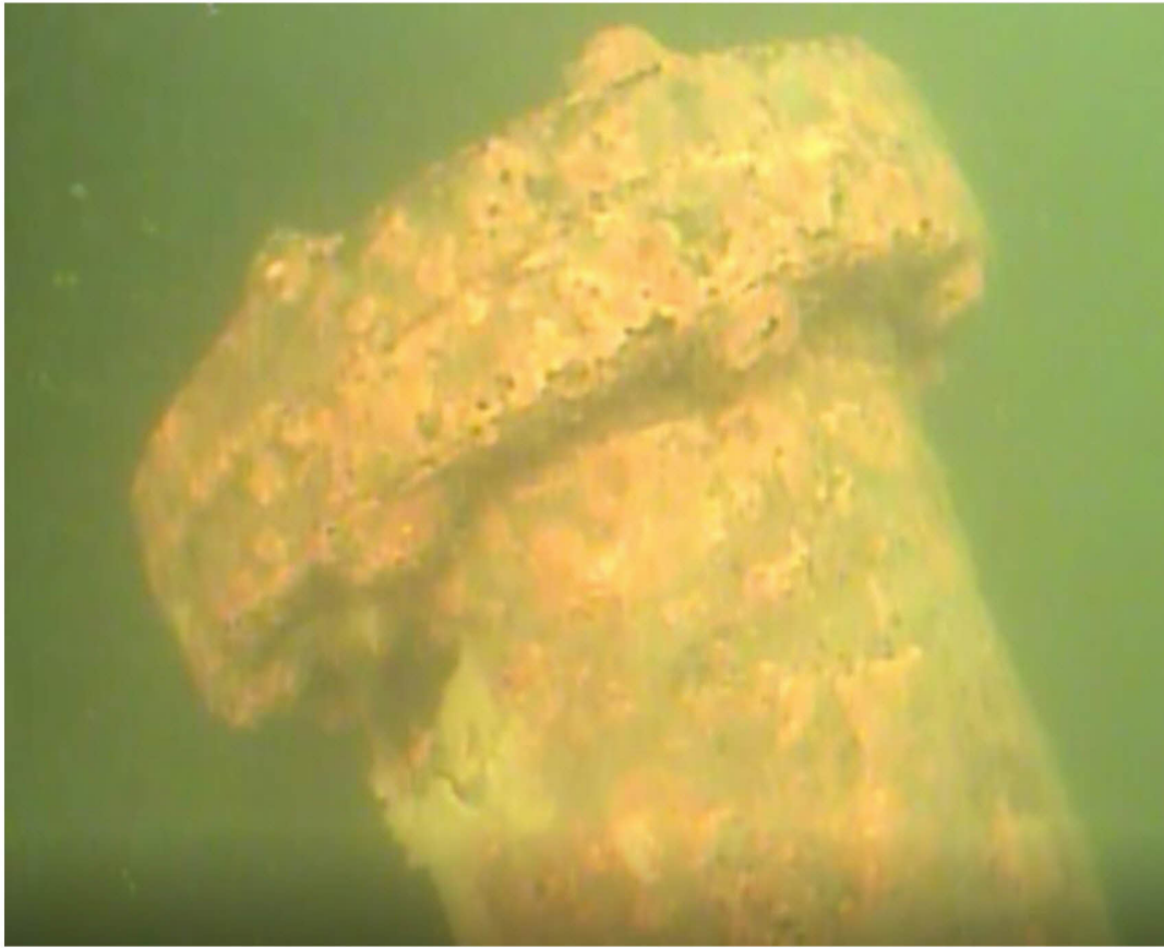
Figure 4- Blind flange and hardware from backside
