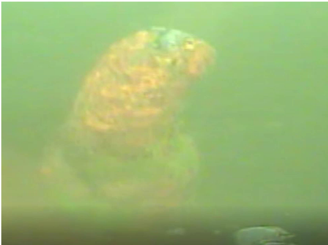
Figure 9- Diffuser #4 during flow test
