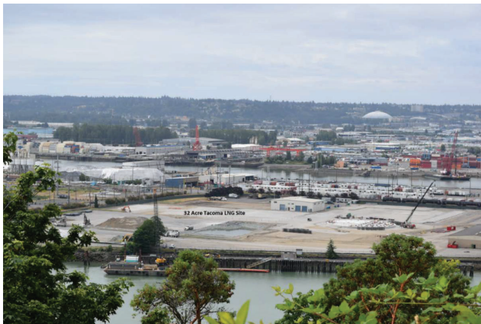
Figure 3 – Tacoma LNG Site, July 2017 (Looking South)
