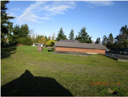
Water Facilities Site
