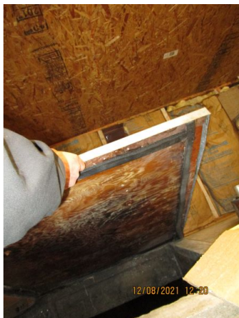
Small Storage Tank Hatch Gasket
