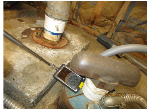
Small Storage Tank Vent
