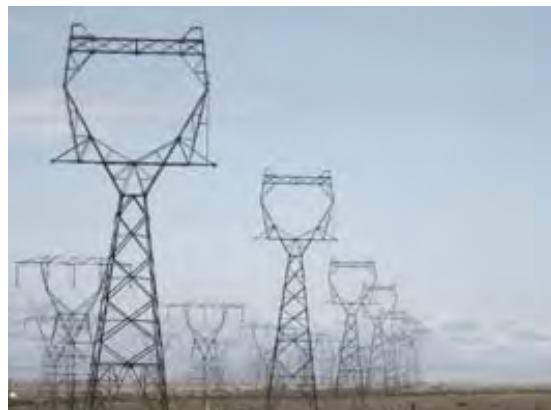
Top: Linemen bolt the top of a banjo tower to its base on the McNary-John Day transmission project. Below: Miles of recently completed towers await stringing with conductor.
