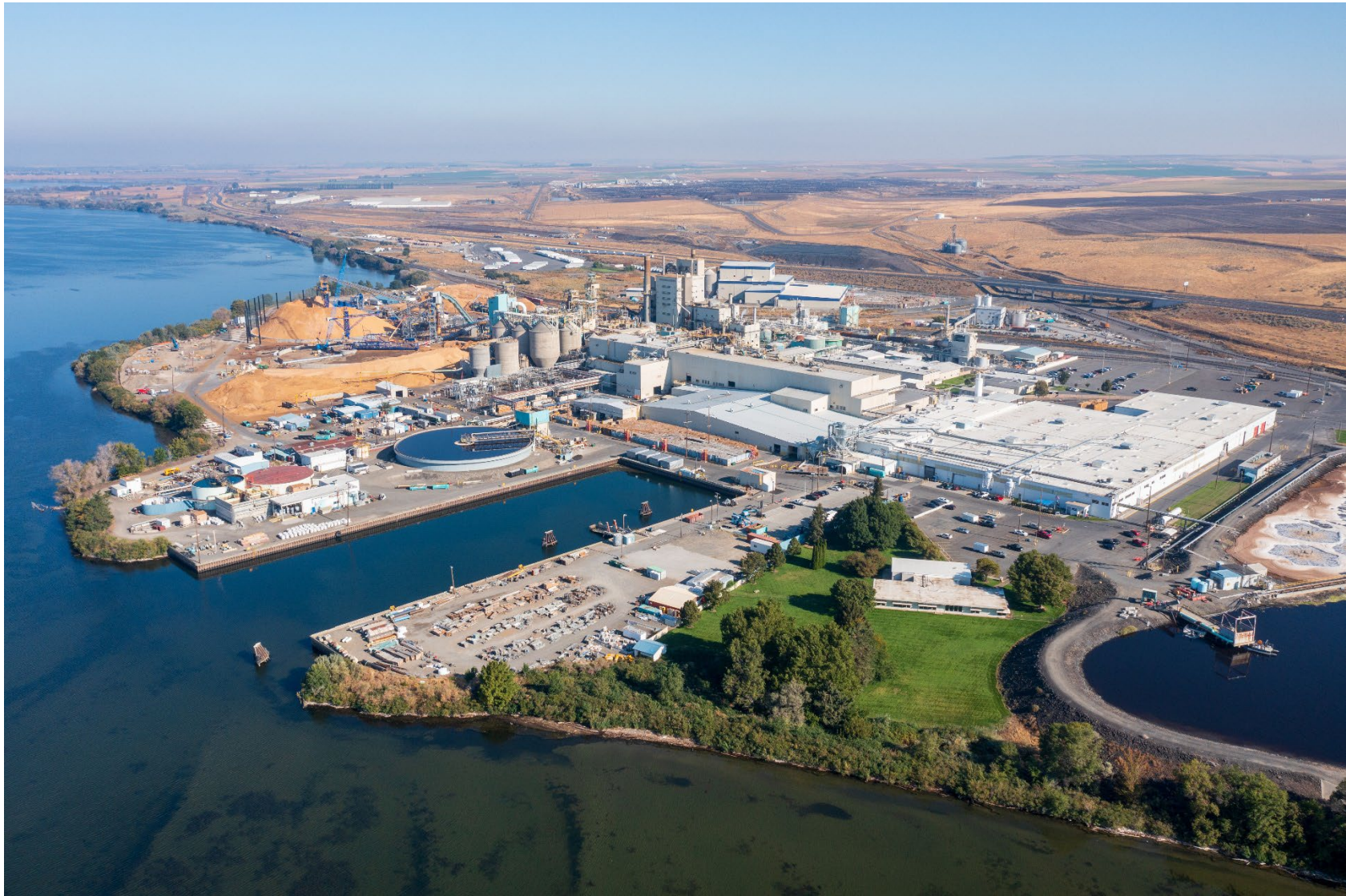
Aerial photo of the Wallula Mill
