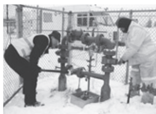
Natural gas crew, 2008.
