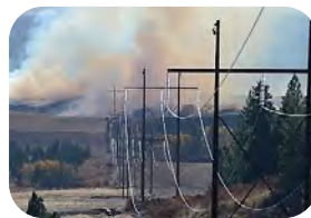
Operations & Emergency Response
