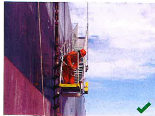
Figure 3.1 - Correct use of PPE
