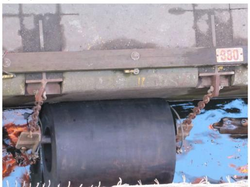
Figure 8. Cylindrical fender on Vanterm berth 5 (Source: TSB)
