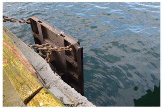
Figure 9. Cone fenders on Vanterm berth 6 extension (Source: TSB)
