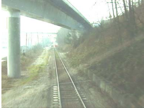
The location of many SkyTrain piers may limit the amount of new tracks that can be constructed between the Fraser River and downtown Vancouver, BC.
