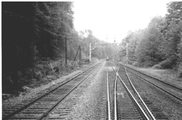
A crossover allows trains to change tracks.
