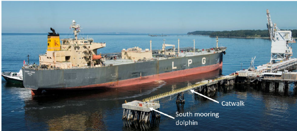
The Petrogas Wharf with a tanker of similar size to the Levant docking starboard side to the wharf. (Source: Petrogas, LLC)
