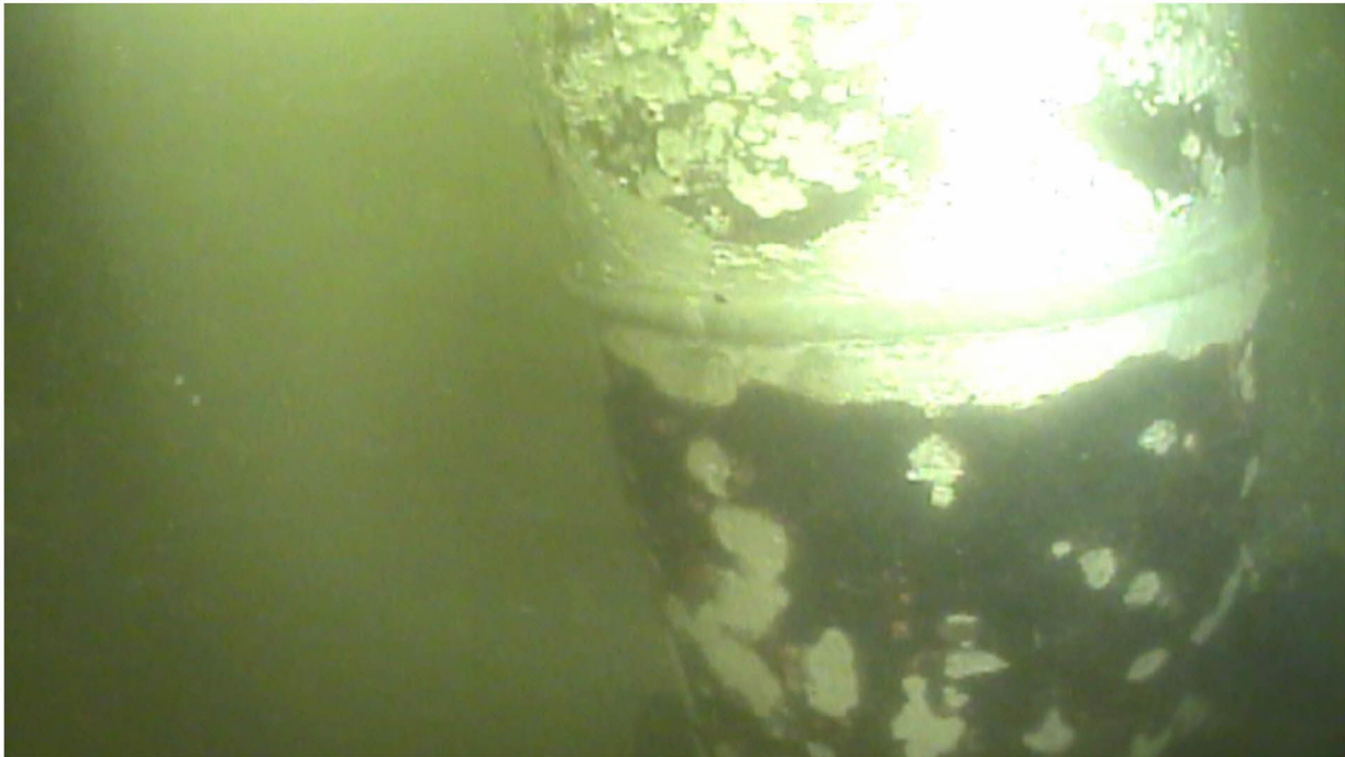
Figure 3- 8” Outfall weld connection in good condition
