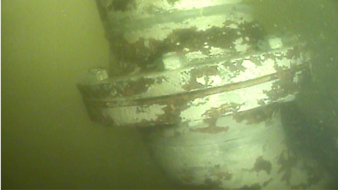
Figure 2 – 8” Outfall pipe flange connection, clean and in good condition
