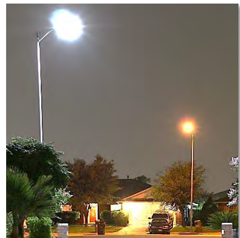
LED (left) vs. Sodium (right)
