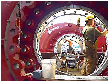
Maintaining a hydro unit
