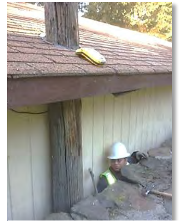
Crews face a variety of unique situations in inspecting wood poles
