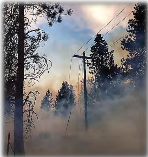
Distribution Line destroyed by wildfire
