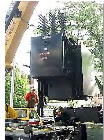
Placing a Pad Mount Transformer
