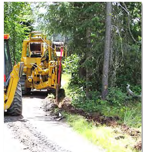
Installing underground cable
