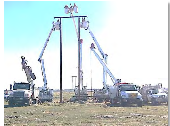
Upgrading Othello transmission lines
