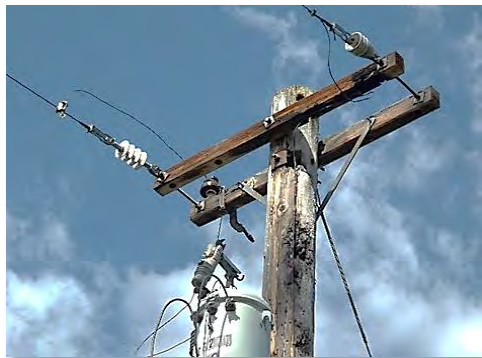
Above: Fire damaged pole Below: Broken crossarm
