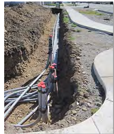
Installing Underground in Coeur d’Alene
