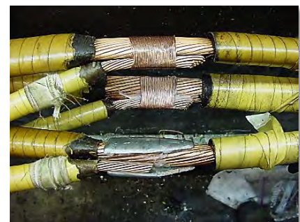
Downtown network crew beginning the process of filling cable with lead to create a solid splice; this type of work is considered an art
