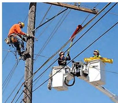
Using a “hot stick” to work on energized lines
