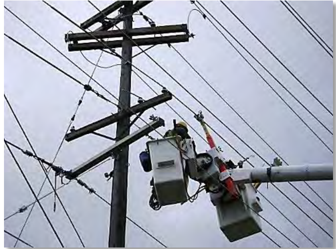
Overhead distribution work
