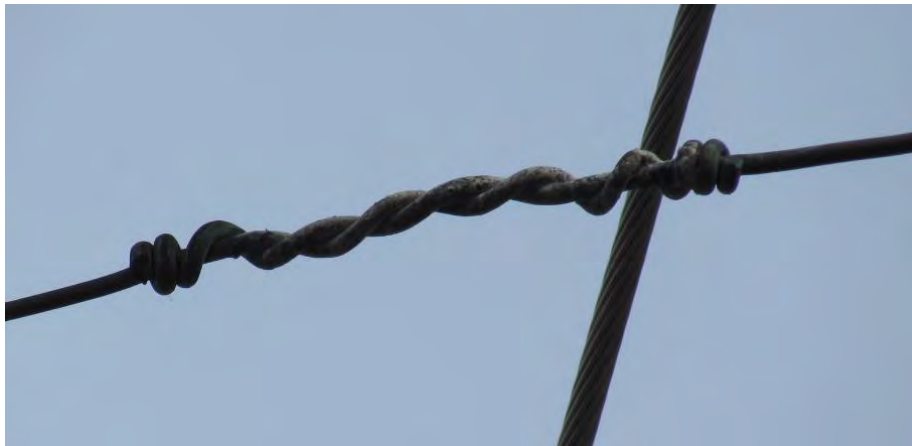
Figure 16: "Western Union" Style Splice
