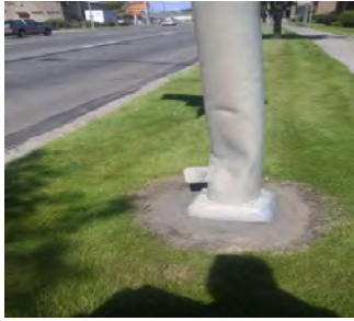
Figure 19: Pole Damage
