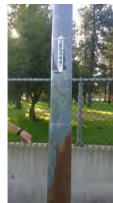
Figure 24: Pole Rusted
