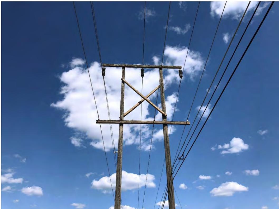
**Figure 33. Three-Phase Primary River Cross at Pole #000053**
