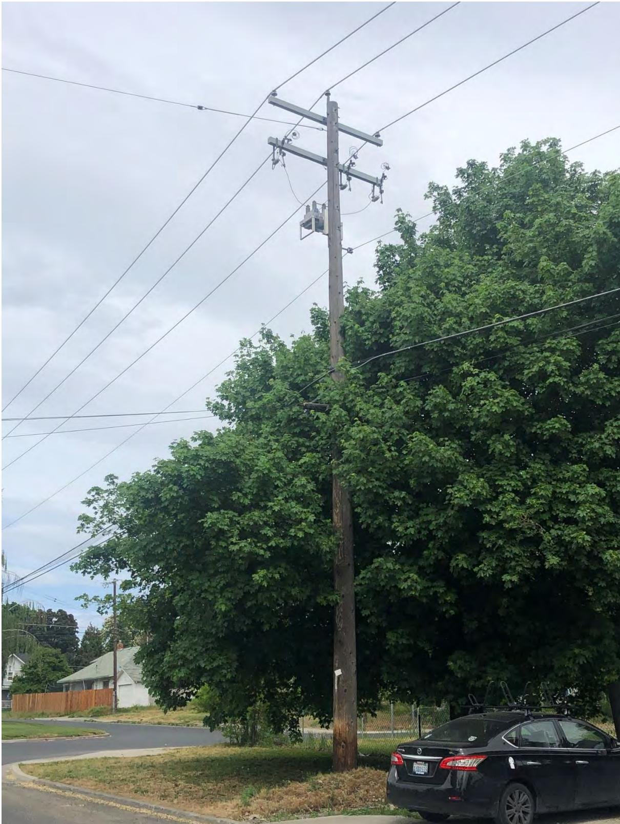
**Figure 24. 600 kVAR 2-Bushing Style Capacitor Bank at Pole #303125**
