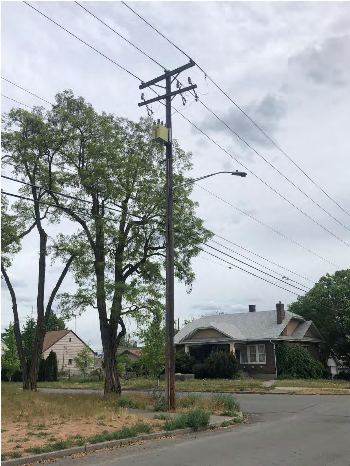
**Figure 23. 600 kVAR 3-Bushing Style Capacitor Bank at Pole #084410**
