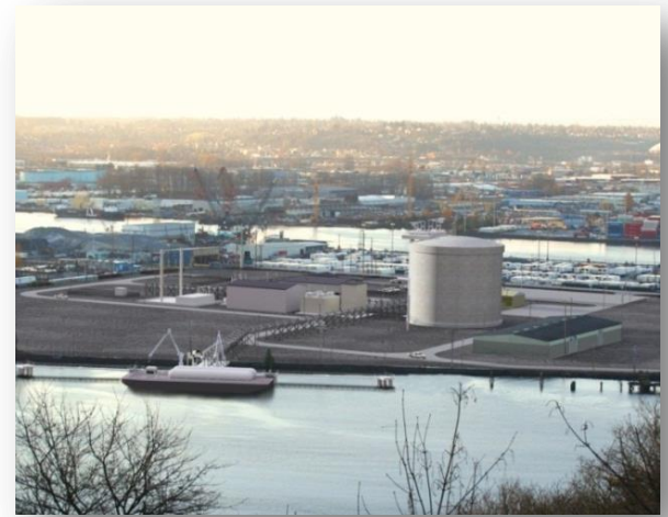
Tacoma LNG Facility in Tacoma, Washington
