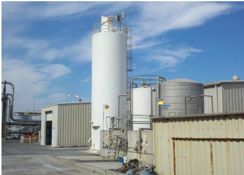
Figure 3: High Pressure Sodium Lighting Outside Demin Building
