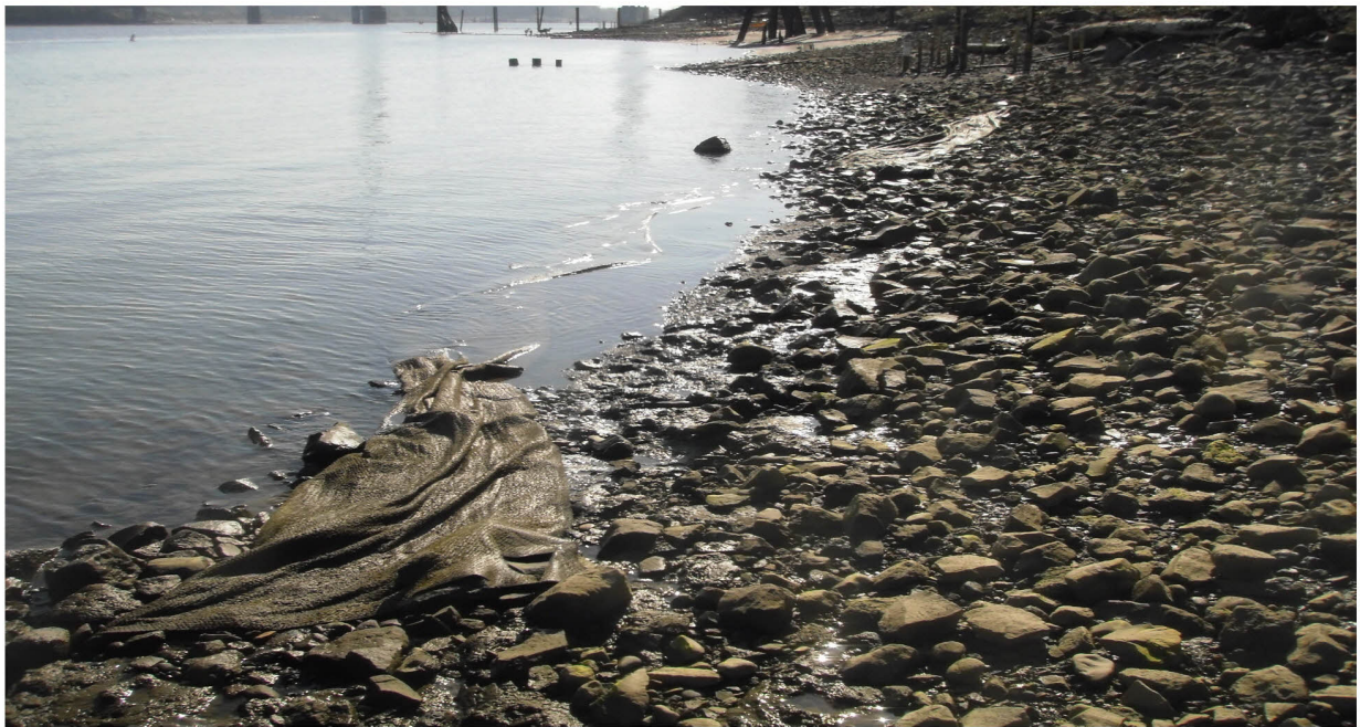
Photo 2 Mat Material Visible at the Downstream End of the Cap Area (3/20/2020)
