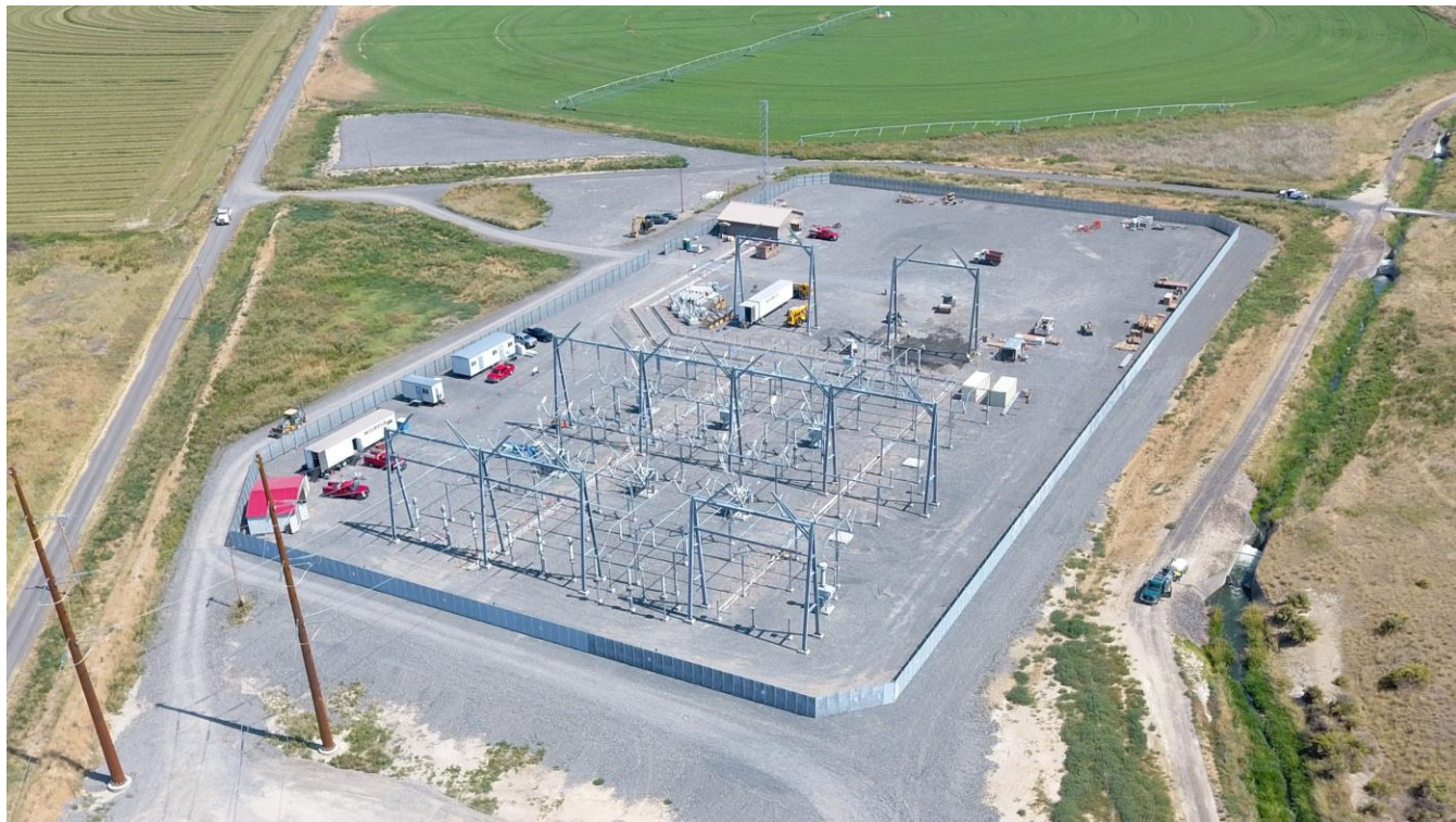
SADDLE MOUNTAIN STATION UNDER CONSTRUCTION
