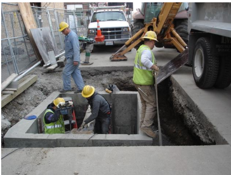
Figure 27, Complete replacement of a badly deteriorated manhole
