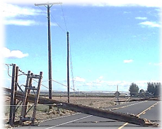
Pole hit by a truck
