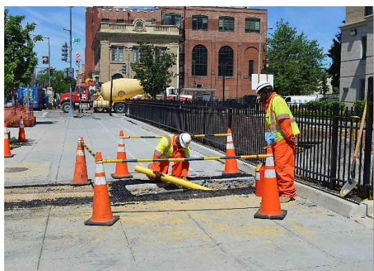
Natural Gas Pipeline Repair in Downtown Spokane
