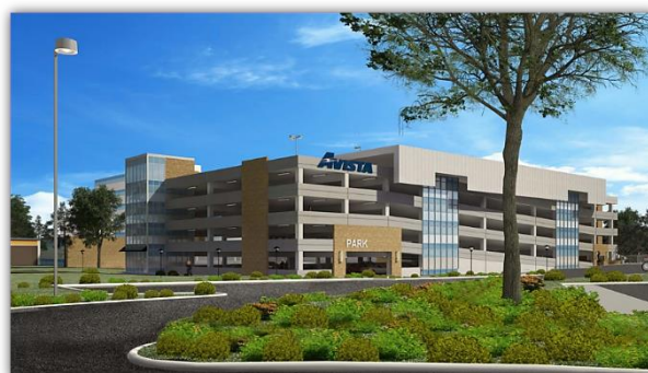
Main Campus parking structure when completed
