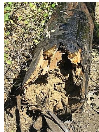
Pole rot causes a failure
