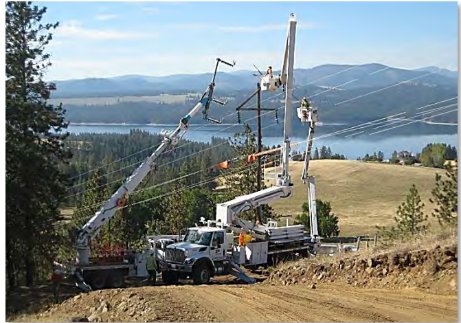
Figure 29. Addy-Gifford Steel Pole Replacement Work
