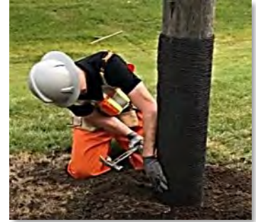
Installing Pole Wraps
