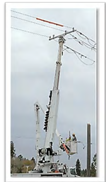
Figure 13. Grid Hardening Work
