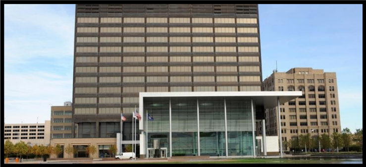
DTE Headquarters in Detroit, MI Source: U.S. Department of Energy
