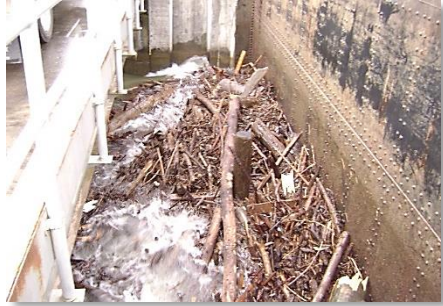
Above: Corrosion on Cabinet Gorge Spillgate #8 Left: Spillgates are subjected to a lot of different damaging factors, including river debris (Spillgate #6)
