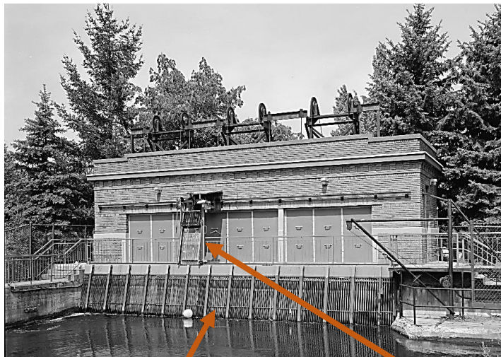
Original Upper Falls trash racks (across the front) and trash rake (above the trash racks)
