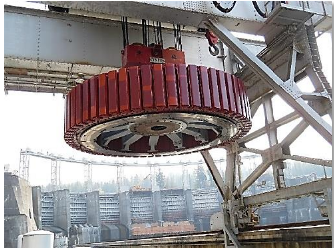
Cabinet Gorge rotor being pulled for maintenance
