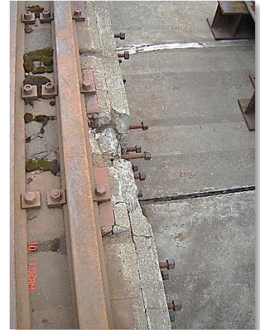
Above: Cabinet gantry crane runway degradation Below: Gantry Crane and runway
