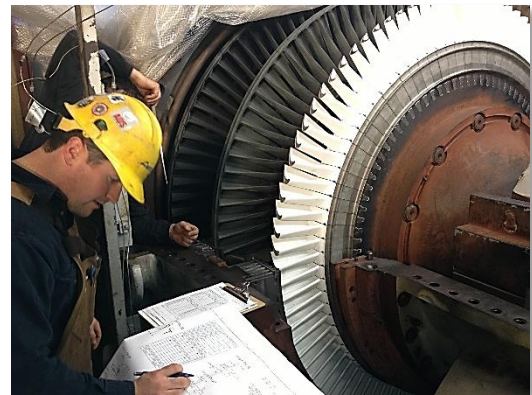
Rathdrum turbine inspection
