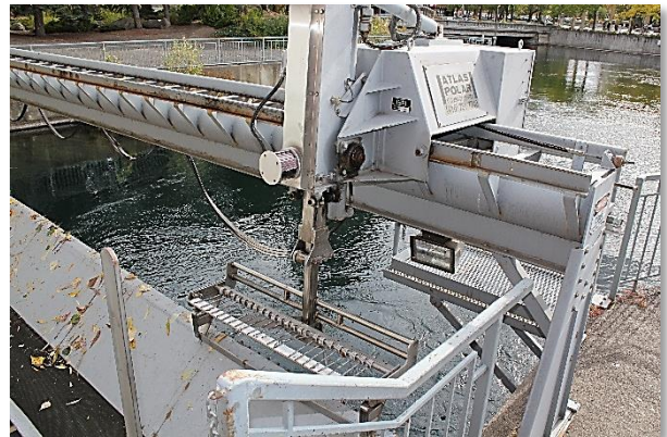
Above: Upper Falls trash rake
