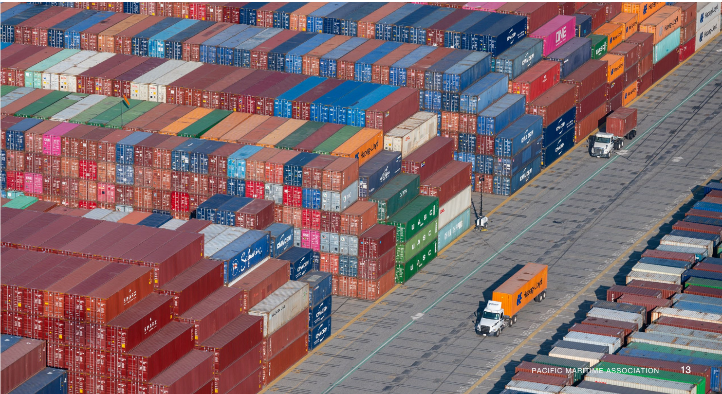
STOR facility at the Port of Long Beach's Pier S.
