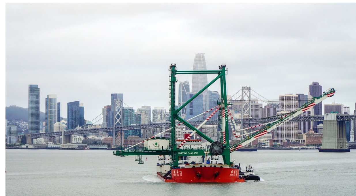
Giant ship-to-shore cranes sail past the Bay Bridge en route to the Port of Oakland.
