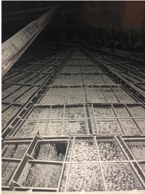
1 Illustration No. 6: Unit 4 Air Preheater Basket Condition
