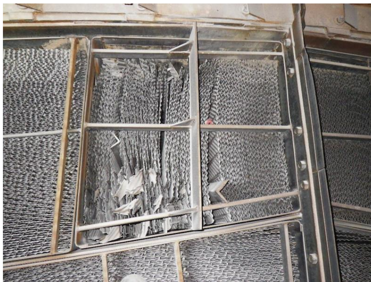
14 Illustration No. 7: Unit 4 Air Preheater Basket Condition
