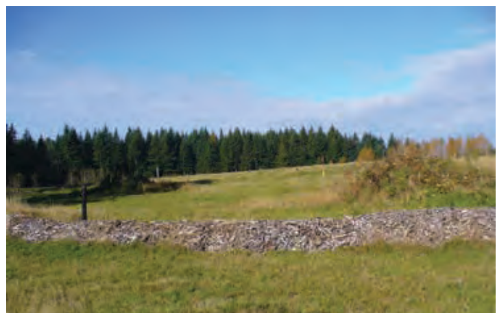
A bioberm at the Cedar Falls closed landfill filters landfill gas
