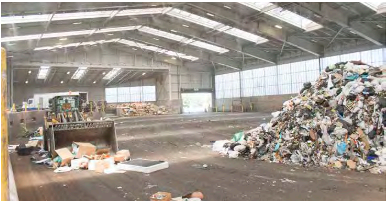
Bow Lake Recycling and Transfer Station
