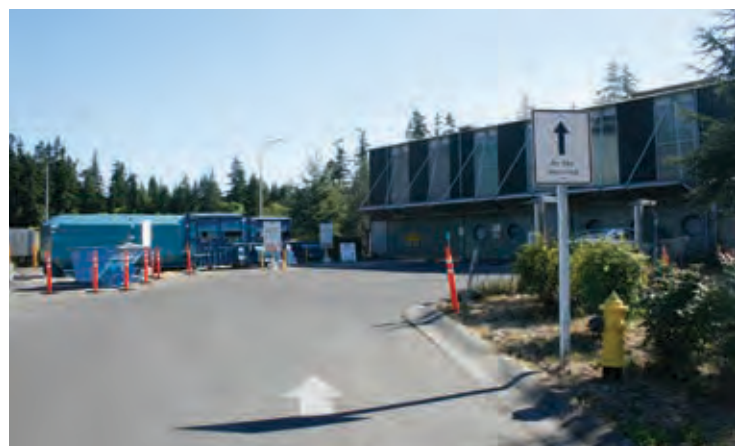
The Vashon Recycling and Transfer Station
