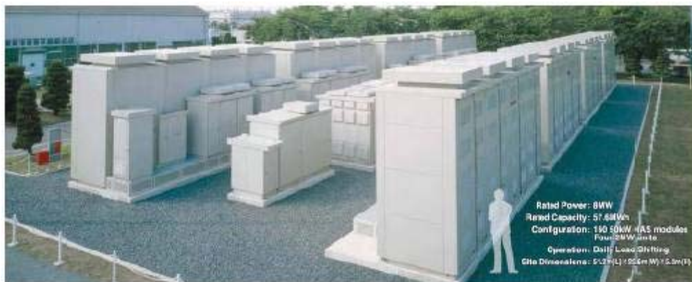
Figure 10 - NGK NAS 8 MW (Japan)
