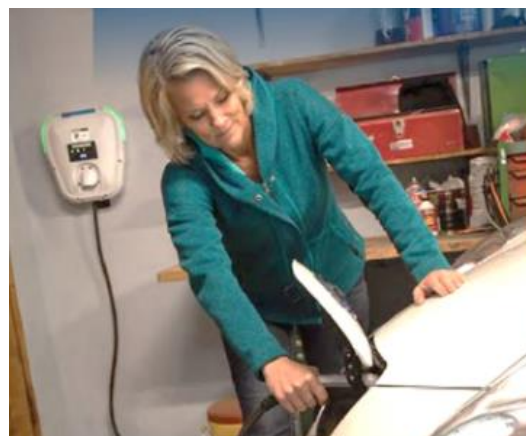
Figure 1: Residential EVSE charging
