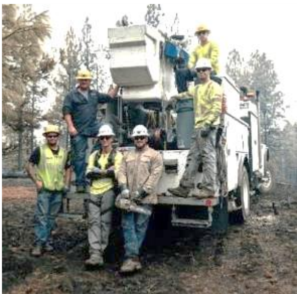
Avista Crews Restoring Power in Medical Lake
