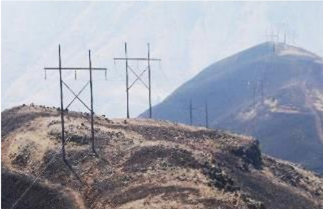
Avista steel transmission poles survive the Snake River Complex Fire
