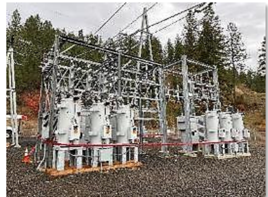
Substation work being completed at the St. Maries Substation
