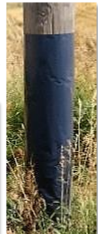
Fire mesh can last more than 20 years and requires no maintenance.
