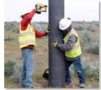
Installing Pole Wraps
