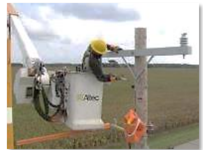
Installing a Fiberglass Crossarm
