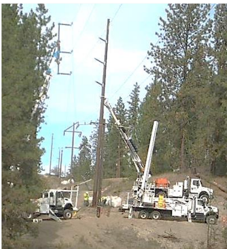
Transmission Pole Replacement on the Addy-Gifford line
