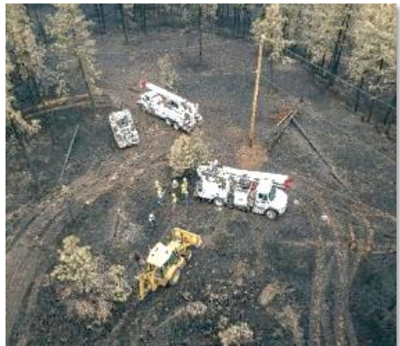
Avista Crews Restoring Power in Medical Lake
