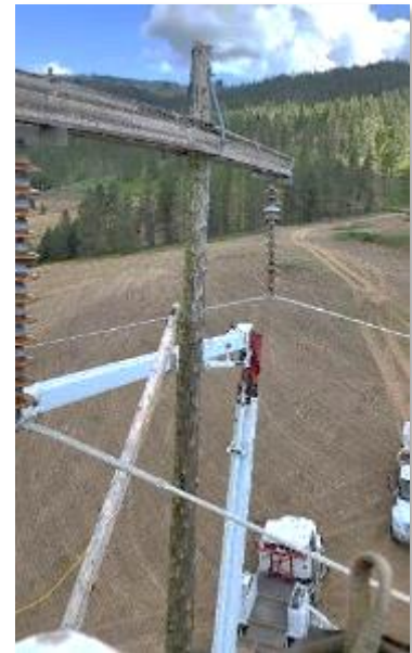
Replacing a bad transmission crossarm
