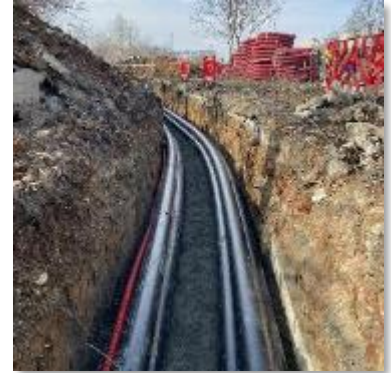
Undergrounding power lines
