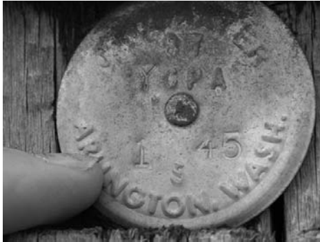
Figure 1 Typical Pole Tag in Pole Gain
