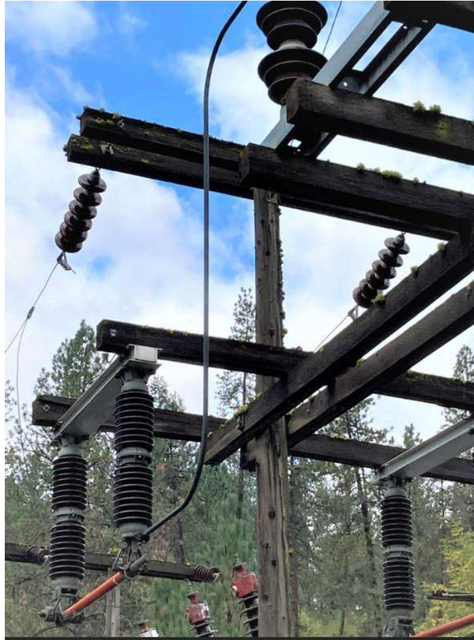
Kooskia Substation with split timbers and moss growing on the horizontal members.
