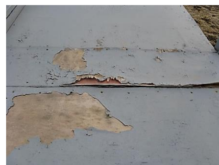
Above: Roof repairs needed
